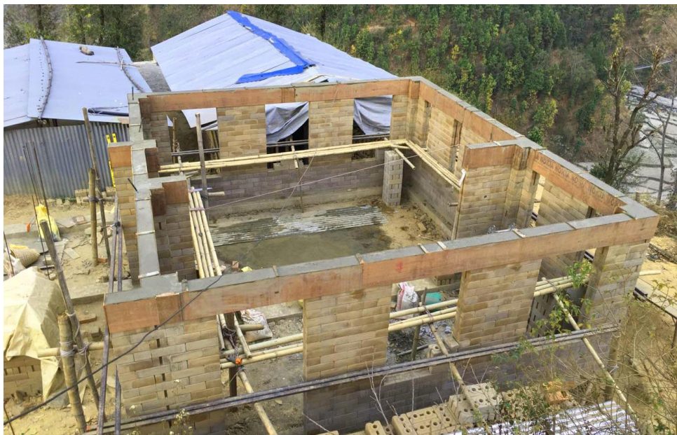
Figure 5: Construction of the first prototype in Sano Bhorle, Nepal (2018)
