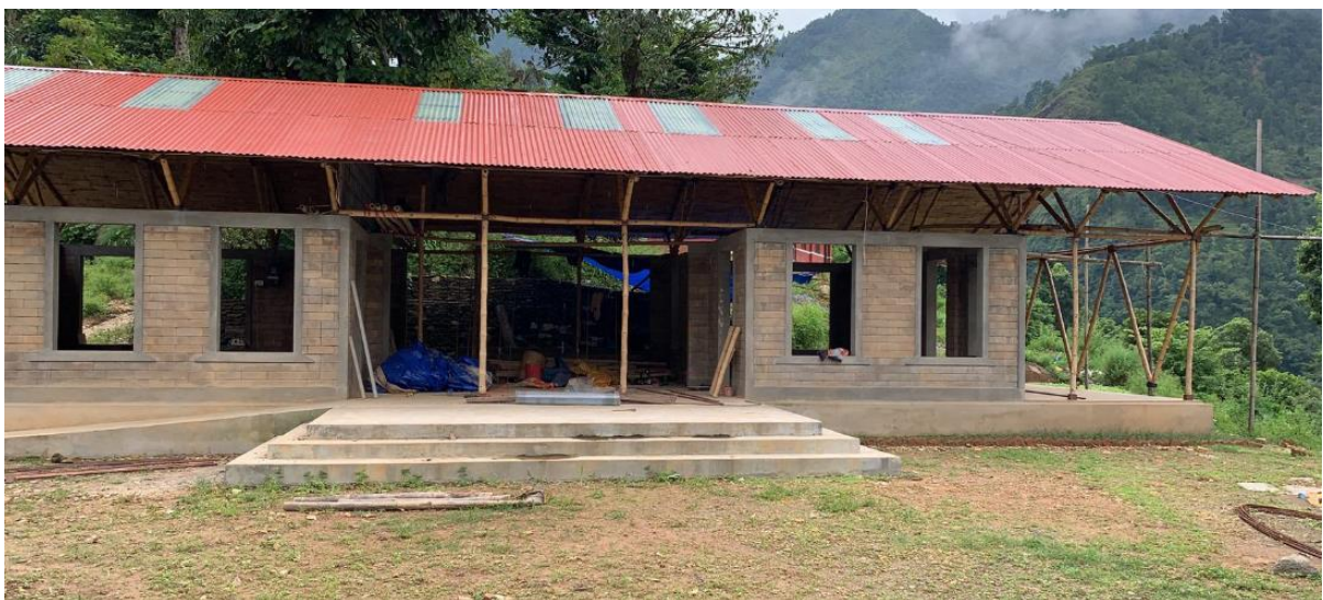
Figure 4: Construction of modular school systems in Sano Bhorle, Nepal
