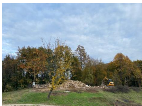
Figure 3: Start of construction
