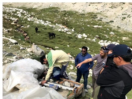
Visit of the local water-supply infrastructure
