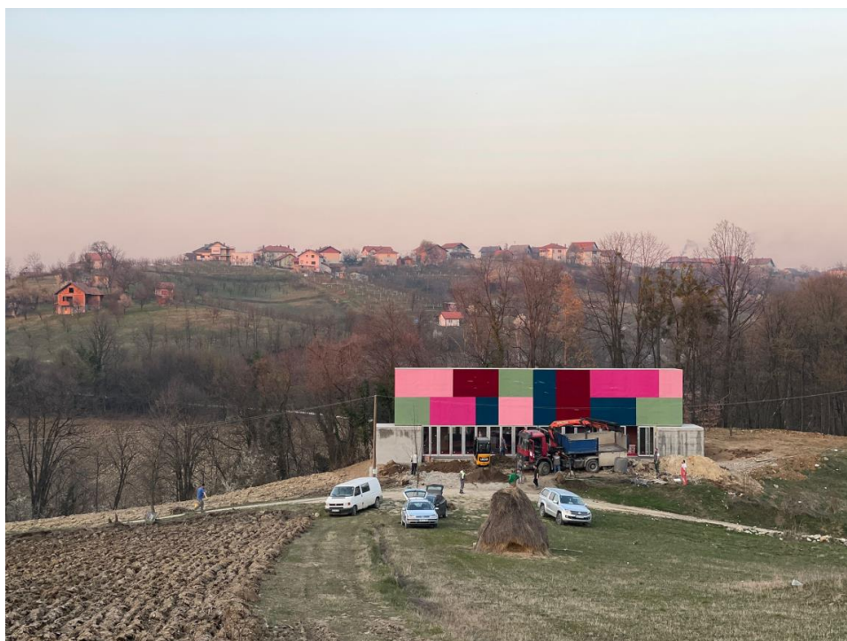
Construction site including the almost finished building
