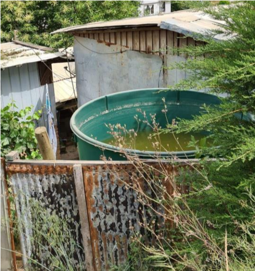
State of current water reservoir tank
