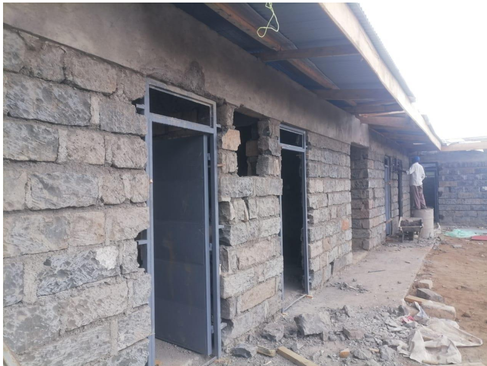
Construction site of new teachers housing quarters
