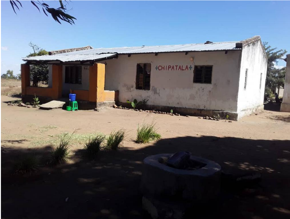
Photo of the old existing clinic
